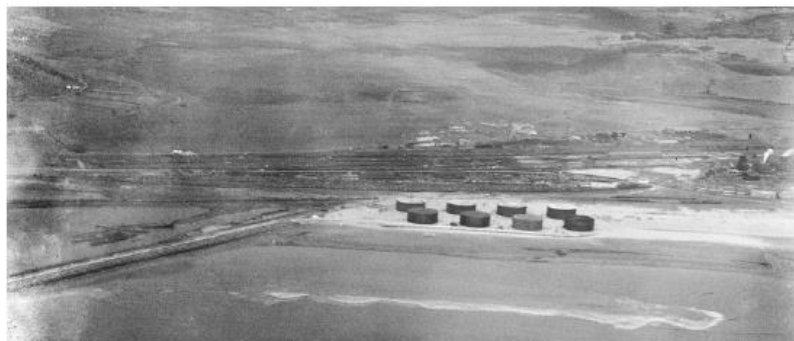
View looking north with the Queens Dock sea wall to the left and start of the petro-chemical tanks to the centre. This area is now the core of the development framework.
