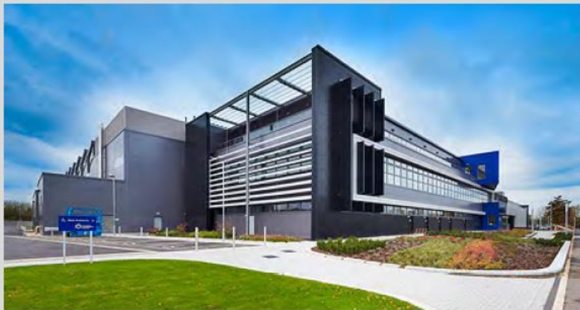
The National Composites Centre at the Bristol and Bath Science Park is a good example of a Research and Development complex with three storey 'active frontage' onto a spine street comprising ancillary offices and legible entrance and a single storey 'supershed' concealed behind.
